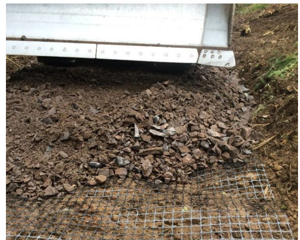
Figure: Appropriate spreading of aggregate fill over RockGrid.
