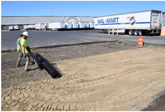
Figure: Manual placement of RockGrid.
