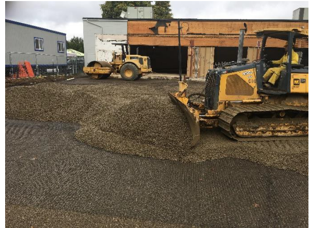
Figure: Appropriate spreading of aggregate fill over RockGrid.
